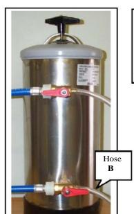
To regenerate the water softener move the top red lever 180°, move the bottom red lever 180°. Water should now start running from hose B, allow the water to run for 30 minutes.
